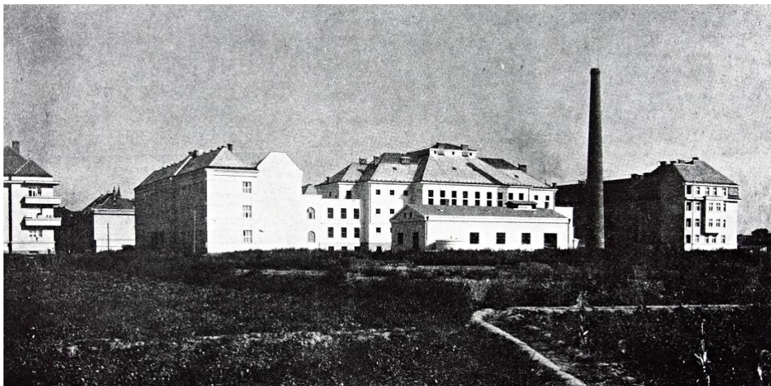
Figure 9: Courthouse – sedria and penitentiary – overall view
